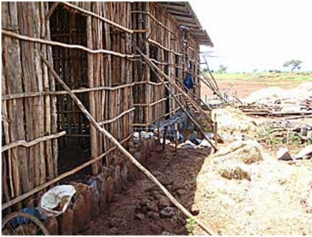
CHIKA-READY: a H4H house under construction in Bahir Dar
