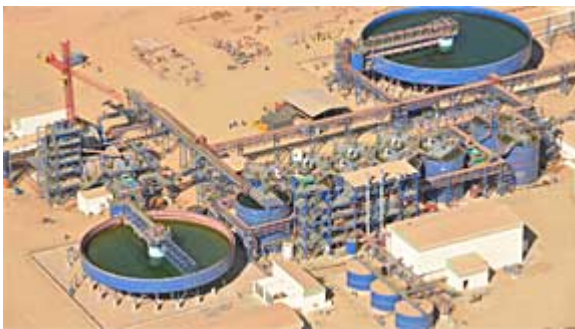
Smelting and production facilities at Bisha
