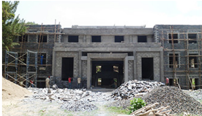
Newly installed façade, June 2015
