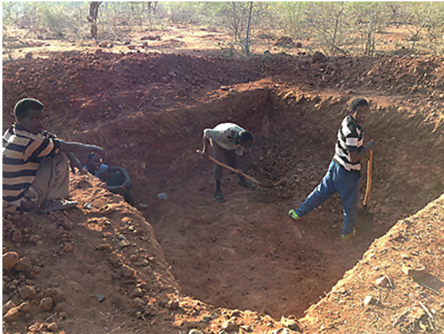
Digging the hole for the Secondary School latrine.
