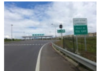
Expressway from Adama
